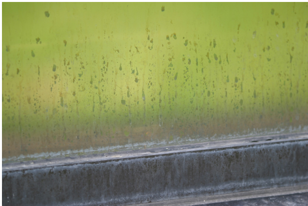
Figure 17: Close up view of silicate deposits on a coated glass surface arising from repeated contact with hard water droplets.
